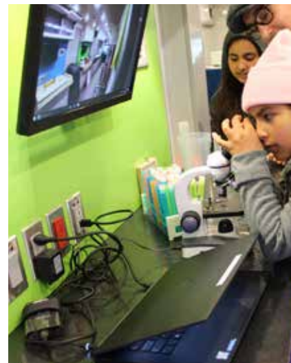
Workstation power receptacles. Red outlet tied to photo voltaic system, gray outlet tied to generator. San Jose Public Library Maker[Space]Ship, CA.
