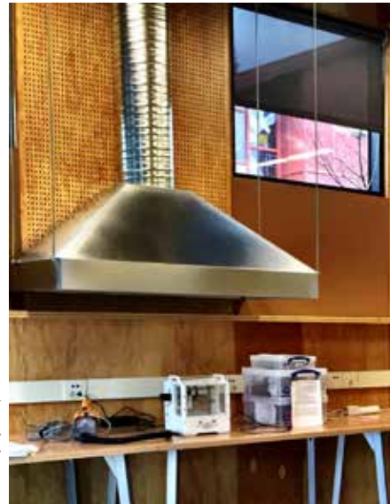
Work counter with Exhaust Hood
