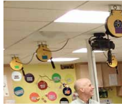
Power reel retrofit, Creativity Lab, Lighthouse Community Charter School, CA.
